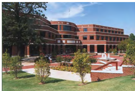
Harding University in Arkansas has 28 Parker boilers installed
