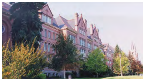
Over 43 Parker boilers are now installed at Gonzaga University in Spokane, WA, with the first unit still in service since its installation in 1963.
